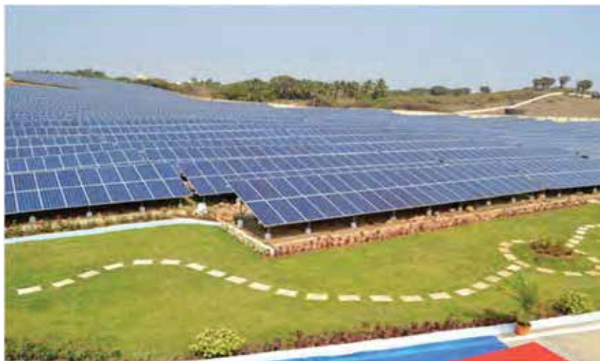
Solar PV Installation, Diu Smart City
