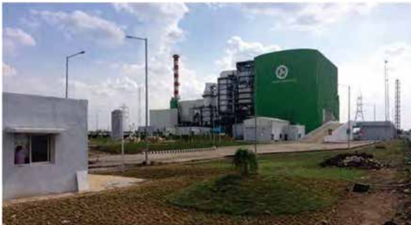
Jabalpur Waste-to-Energy Plant on PPP mode
